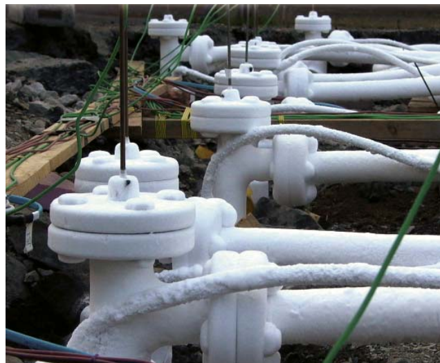
The soil freezing system in operation
