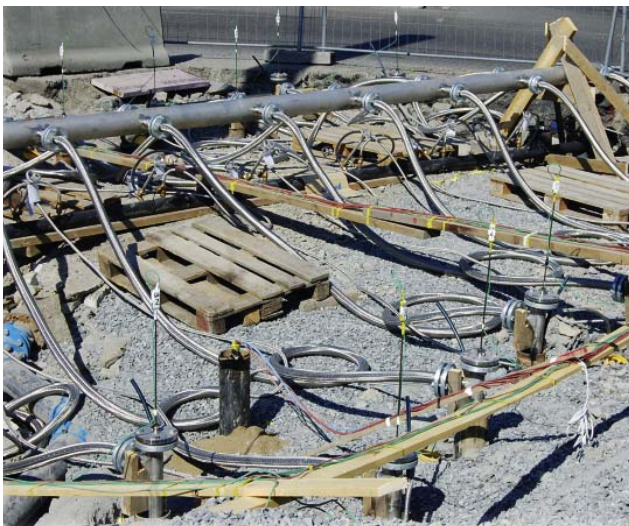
The soil freezing system under construction
