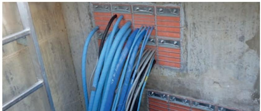
**RGG** frames and the flanges of the **Counter frame** are screwed into the wall (fig. 6). A Lycron sealing strip should be used between the wall and the flange to provide a gas tight seal. The galvanised counter frame is available with three different standard depths, which are suitable for the most common wall thicknesses, see below.
