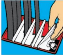
**3** To prevent the blocks from falling through during horizontal installation, fit all the stayplates and the compression plate first. Check the RG plan to make sure the cables are positioned correctly.
