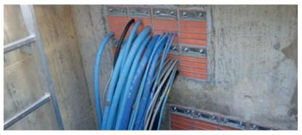
**RGG** frames and the flanges of the **Counter frame** are screwed into the wall (fig. 6). A Lycron sealing strip should be used between the wall and the flange to provide a gas tight seal. The galvanised counter frame is available with three different standard depths, which are suitable for the most common wall thicknesses, see below.
