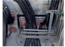
**RGP** and **RGPO** frames are installed on one side of the wall when normal demands are made for fire safety, (see fig. 9.) When the satety demands are particularly high two RGP frames are installed back-to-back (fig. 10). RGP can be installed in drilled or cast holes, or in a pipe that is cast in or bolted. Casting is made easier if MCT Brattberg casting forms are used, see picture.
